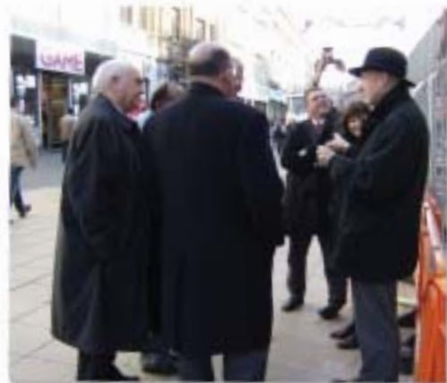
LSEP Board members checking on the progress of work in Leicester City Centre.
